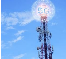
RF and Wireless Communications
