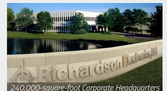
240,000-square-foot Corporate Headquarters
